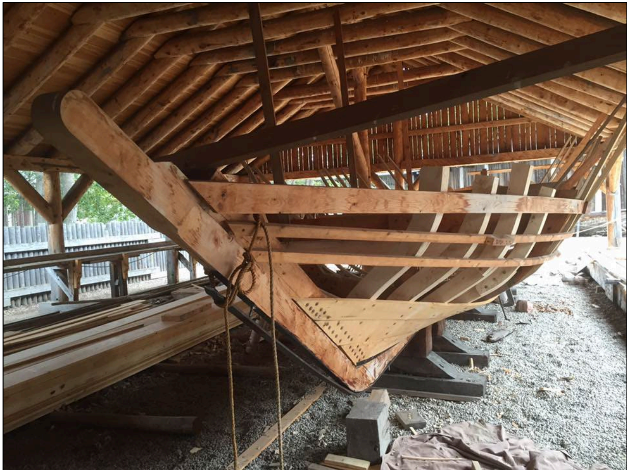
Figure 4-6 York Boat with the first strakes attached at the bottom of the boat. The Iron Stem Plate or strip can be seen, although it is not yet attached.
